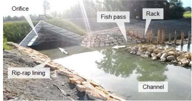
Figure 13: Structures constructed on the Aire River as defined on the physical hydraulic model. A hexagonal orifice and a rip-rap channel bank lining were adopted upstream from the latter.
